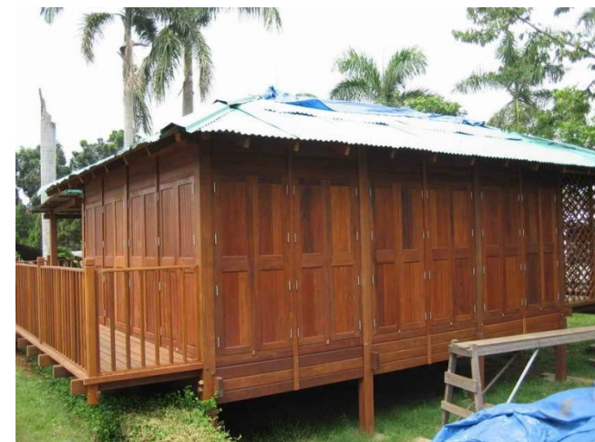
Complete Assembly of ifil wood upper floor, in Indonesia.
